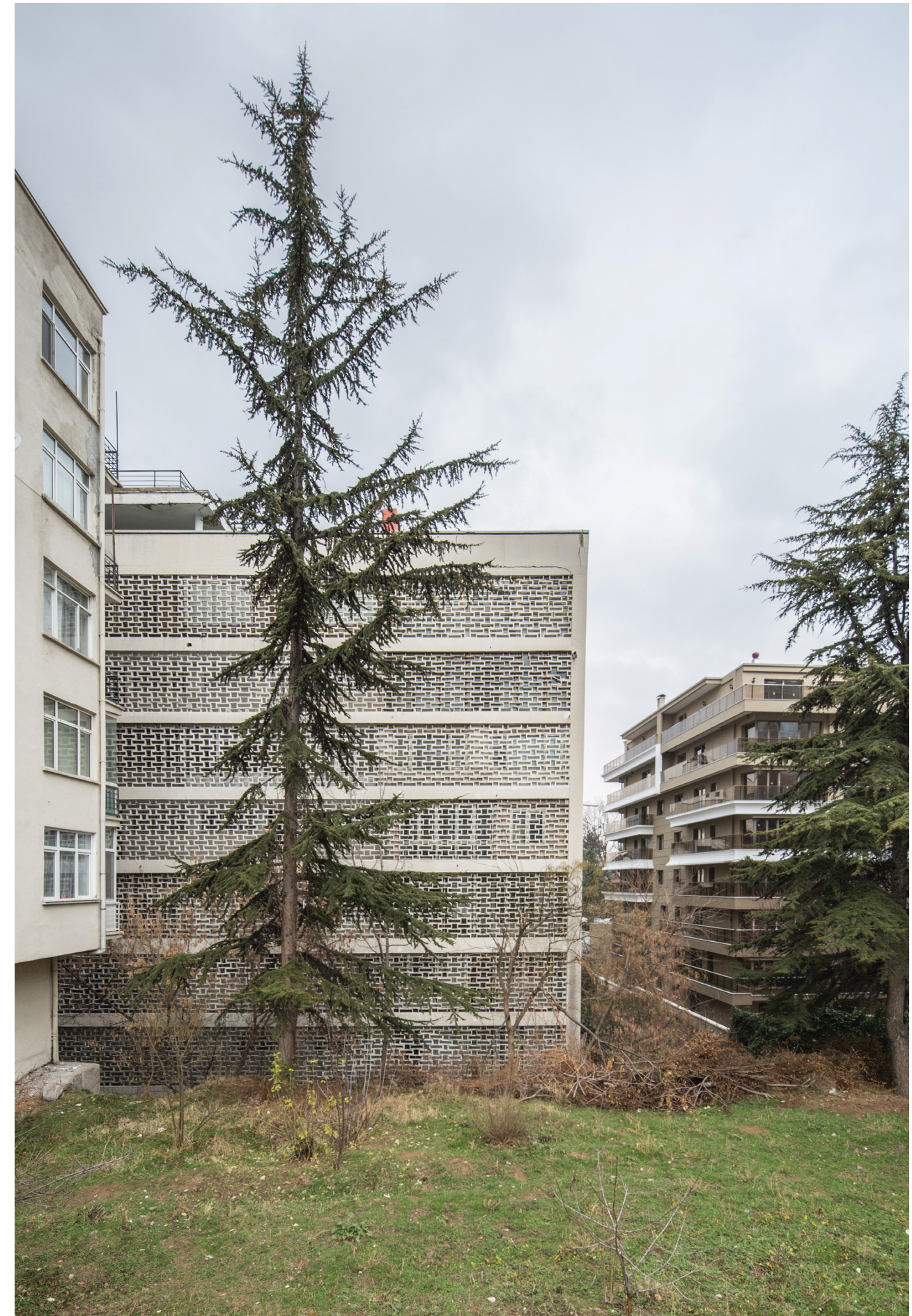
Southern (rear) façade of the building with brise-soleil. Photography: Duygu Tüntaş, 2019
