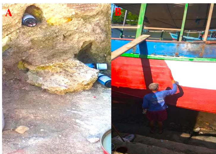
Figure 5. (A) Dam compound used as a biocidal agent to enhance the action of paints; (B) fisherman performing maintenance on the painting of the vessel on the river bed, with biocidal compound mixed with paint. Source: Author (2022)
