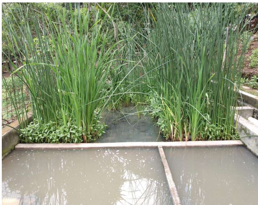
Figure 2. Single-stage wetland plant.
